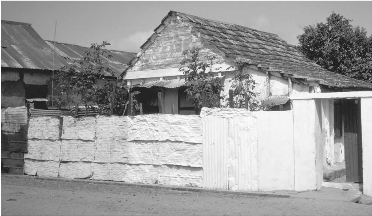
A house in Sokone, Senegal, has protected privacy with a painted metal fence.
